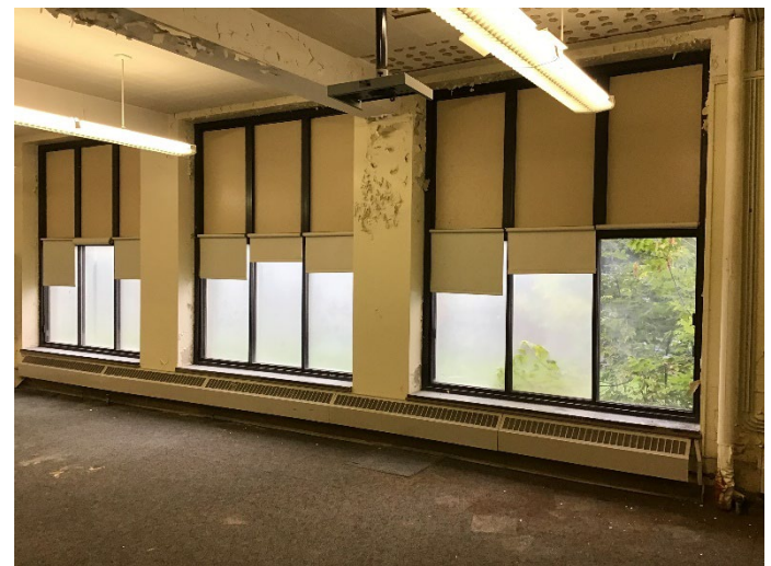
Interior Kensington from 2020 PMC FCA walkthroughs. Building is being vacated.
